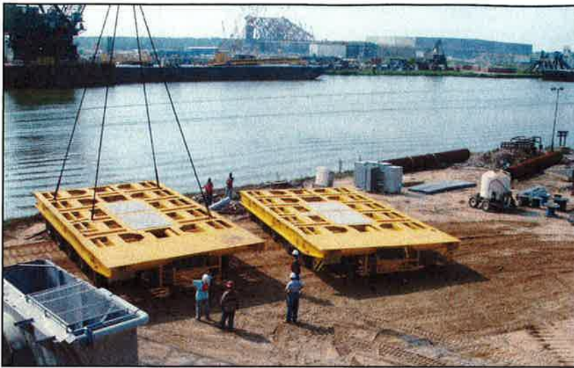
The two 226 tonne transporters have been saved from the wreck of the New Orleans harbor after Hurricane Katrina.
